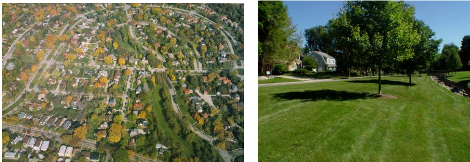
Figures 2a and 2b: The central organizing feature of Washington Highlands is its linear greenway seen as a green ribbon in the aerial view (left), and also in the photo on the right. The curving boulevard bounding the neighborhood (left, at top) is said to have been inspired by the outline of a Prussian soldier’s helmet, as the designer was German-born. (aerial photo by Jeff Voelz) RA ground photo
