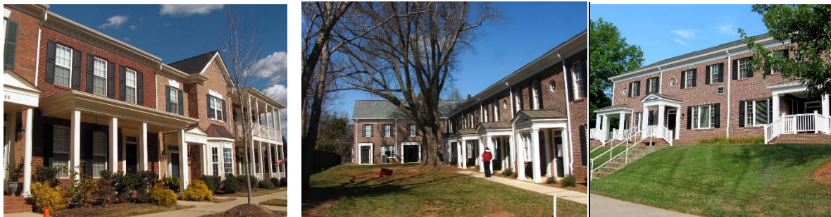
Figure 9-15: The developer of the St. Albans infill neighborhood (left) complied with Davidson's wishes that a number of affordable units not only be provided, but also be integrated physically and not set apart. The design solution was to insert them between market-rate units in townhouse formations, shown above, as was also done at Wyndcrest, noted later in this chapter. In 2006 Davidson College built eight units of attached affordable homes for staff and faculty in an L-shaped building bracketing a small neighborhood green with a large willow oak tree (center). The other side of one of the two wings faces Main Street, with a modest front setback (right).. Ultimate plans call for a second L-shaped building to create a quadrangle and a courtyard. Source: Marguerite Williams (left), Kris Krider (center and right)
