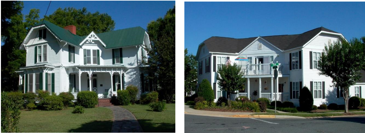
Figure 9-13: The six-unit residence (left), built on Park Street, was modeled on an older house on Jackson Street-(right), whose owner allowed the Davidson Housing Coalition’s architects to measure it to create a multi-family house similar to a large single-family home. This design was used twice at the Bungalows, on opposite sides of the street, creating a dignified gateway to this moderate-income neighborhood. It has also been used once on Potts Street. Source: Kris Krider (both)
