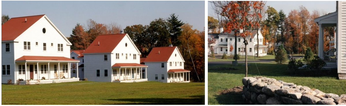
Figure 20-10.2: The rear elevations of these three gable-ended homes present a formal side to the central green, with back porches designed to resemble front porches. The other sides of these deep buildings extend back to the street to encompass additional dwellings in the New England “connected farmhouse” style. Stone walls (right) were relocated and rebuilt to maintain the rural character of this new hamlet setting. Source: Charles Tashima
